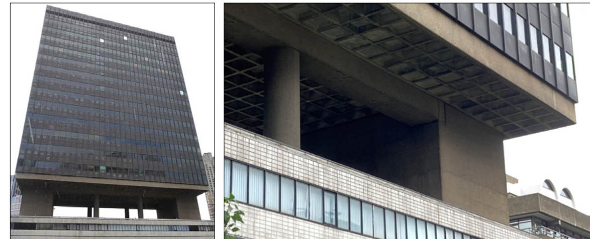
Figure 4—3 Bastion House Tower showing transfer structure above the podium of the Museum of London which is exposed to carbonation and at risk of disproportionate collapse.
